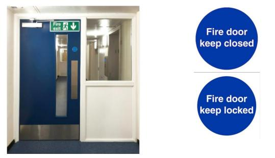
Some doors can be held open with a specifically designed magnetic closer, but these turn off allowing the door to close if the fire alarm is operated.
